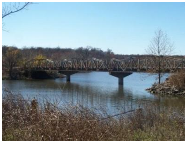
Bridge over Murray Gill Lake
